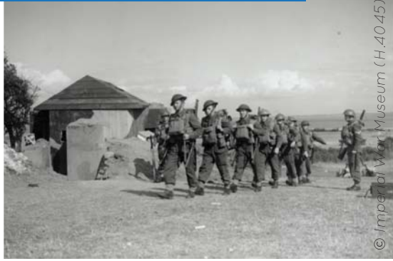
An infantry pillbox camouflaged with a false roof, paint and piles of earth to deceive enemy planes.
